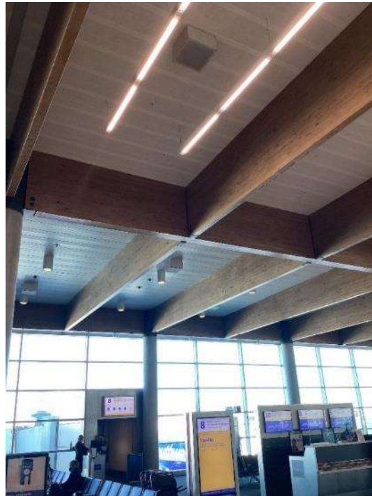
Image 4: Typical Lighting in Concourse
