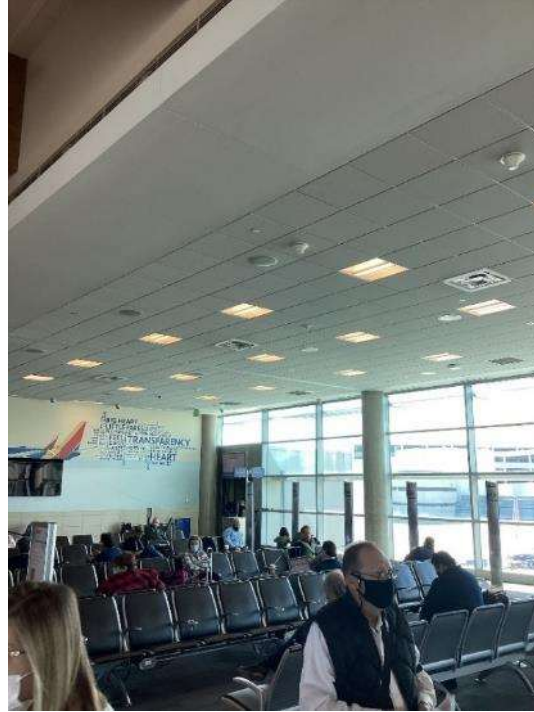
Image 5: Typical Lighting in Concourse (2)
