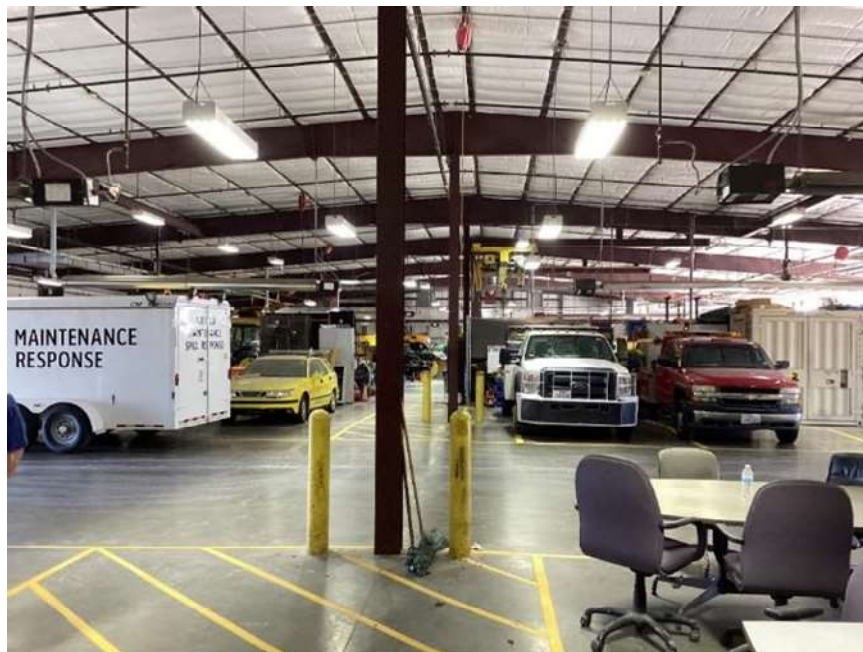
Image 17: Airfield Maintenance Garage Building
